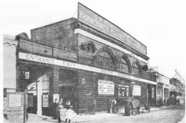
Leslie Green's station building in c. 1910
